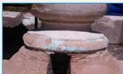
Fountain location of historic plumbing
