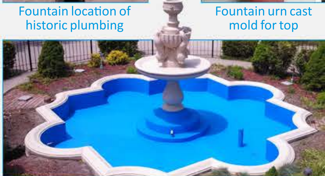
Civic Center Fountain after repairs
