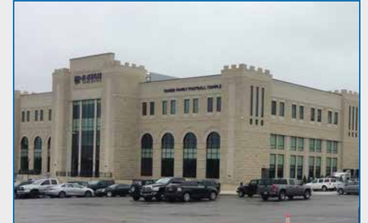
Completed north end zone renovations at the Kansas State University Vanier Football Complex.
