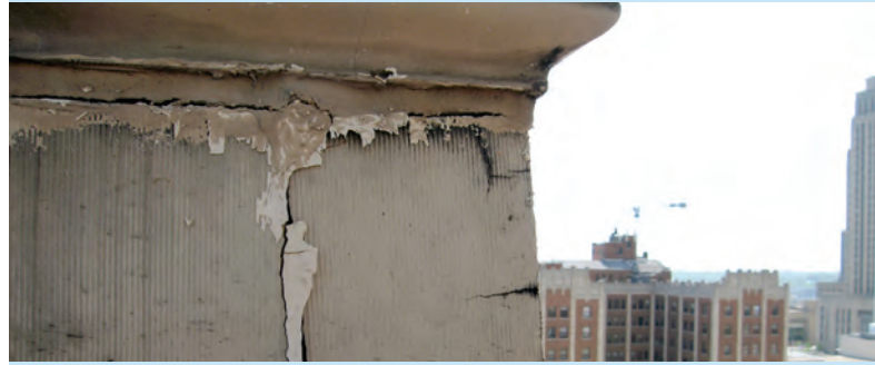
Terracotta ready to cut loose that could be improved with Tuckpointing
